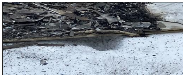
Figure 4 – Melted EPS insulation below the cement-bonded particle board in test 3 where the fire propagated below all the PV arrays. [12].
